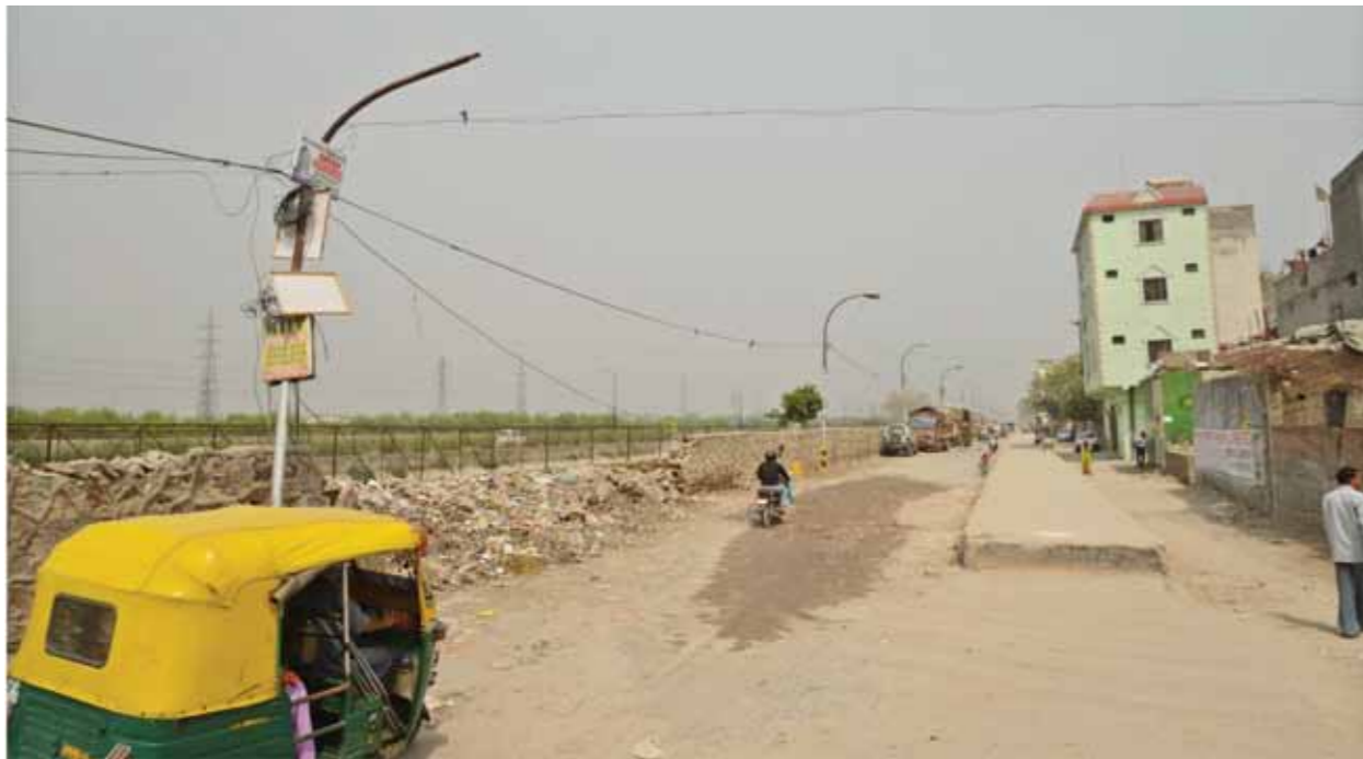
Existing road along canal with garbage dump, undesigned road section, New Ashok Nagar built edge with area to be demolished
