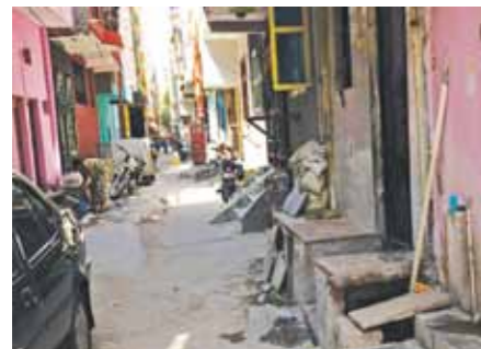
Existing condition of 4.5-m-road
