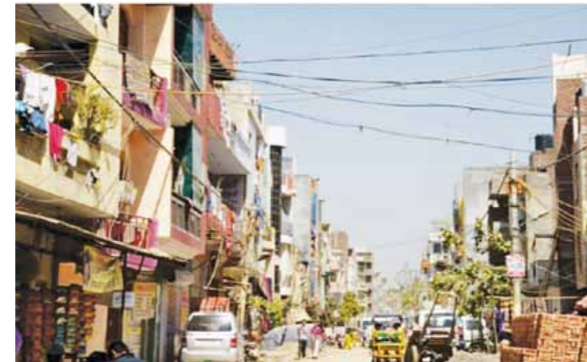
Dangling electric wires
