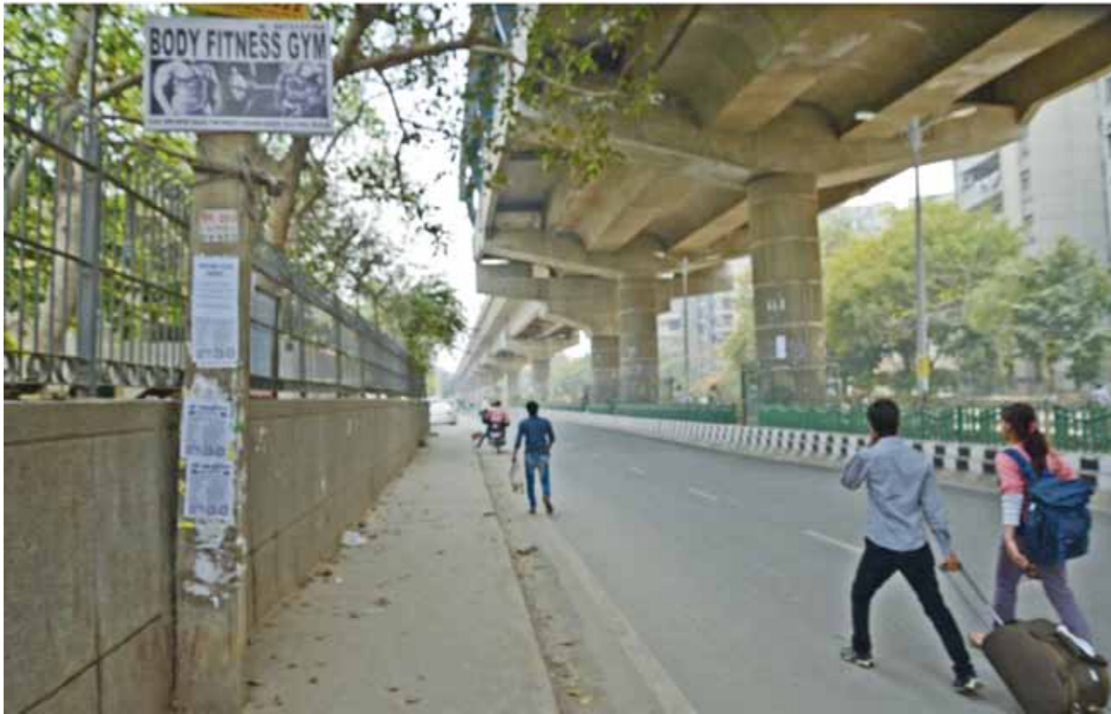
Existing main road with no demarcation of space for pedestrians, non-motorized vehicles, parking
