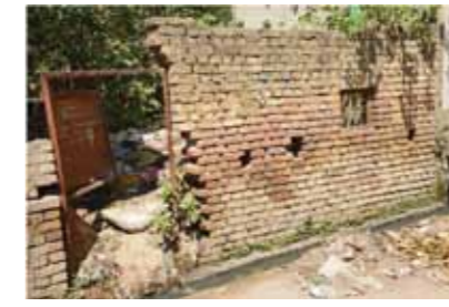
Condition of vacant plots
