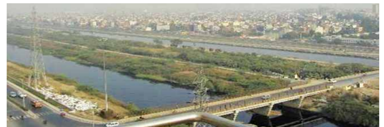
The built edge of New Ashok Nagar overlooking the Hindon Canal & Ghazipur Drain
